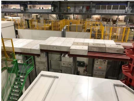
*Figure 3: H4 (NP04) Beamline magnet support blocks*
