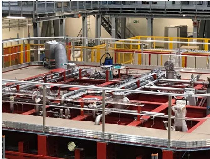
*Figure 2: ProtoDUNE-SP roof cable trays installed*
