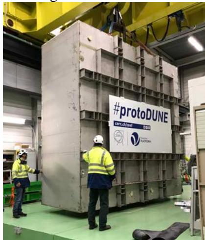
*Figure 1: ProtoDUNE-DP cold box installation in Building 182*
